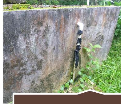
Damaged pipes
